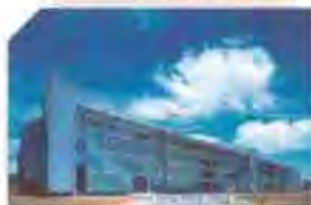
The suspended double glazing facade of the BPO building
